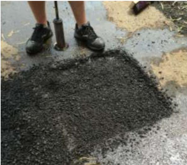
COLDMIX POTHOLE FILLED AND COMPACTED IN TWO LAYERS
